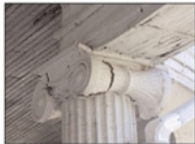
Before and after: parts of the woodwork were replaced with custom milled replicas.
